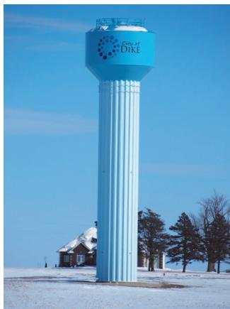
The City of Dike officially connected to CIWA on November 1, 2014, upon completion of a new 300,000 gallon water tower and 10" transmission main upgrades necessary to serve the city.
